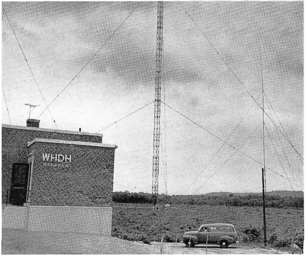
Effective 1/4 wave vertical of W1TOP is shown in above photo behind WHDH station wagon.
