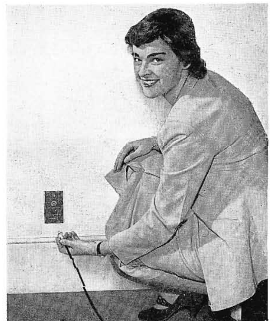
▶ Wall outlets provide the final link of the distribution system. The television receiver is ready for operation as soon as the cord is plugged in.
