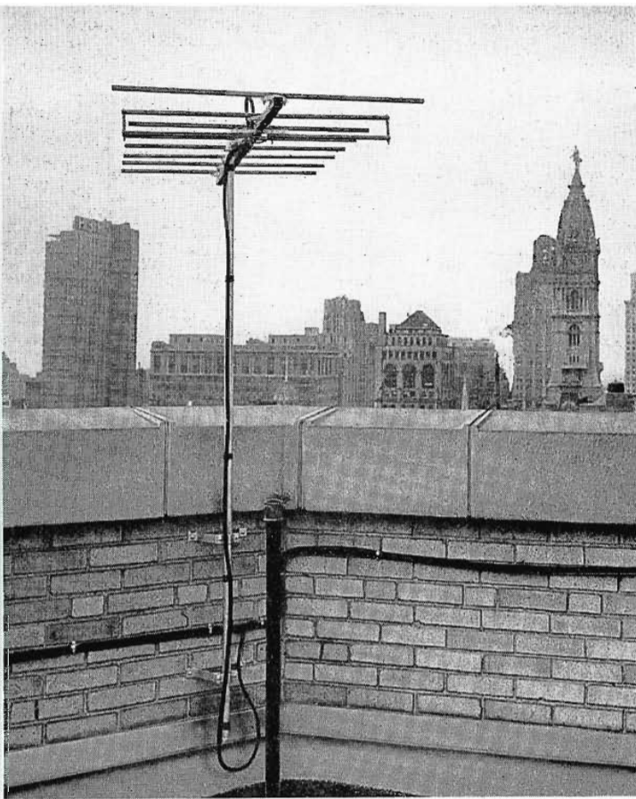
The RCA Television Antenaplex array looms above the 20-story hospital. The hospital is the first in the world to provide patients and staff with this multiple-outlet RCA master television Antenaplex system.
