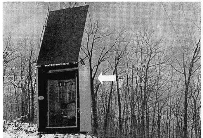
This special RCA Community Television Antenaplex Amplifier greatly intensifies the signals picked up on top of Sharps Mountain—assuring excellent reception in Pottsville homes.
